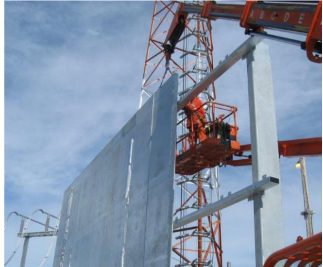
Acoustic DuraBarrier® being installed next to loud machinery.
