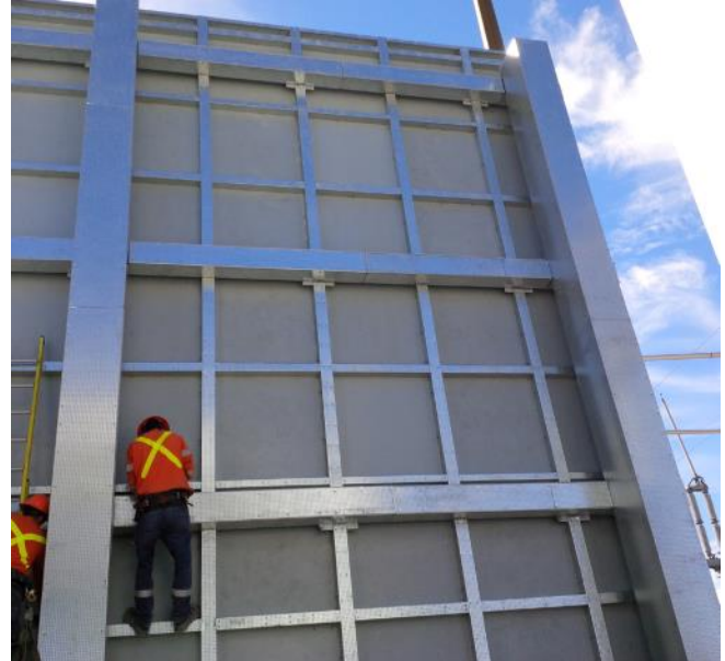
A Ballistic DuraBarrier® installation with girt protection.
