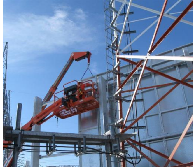
DuraBarrier® module being installed.
