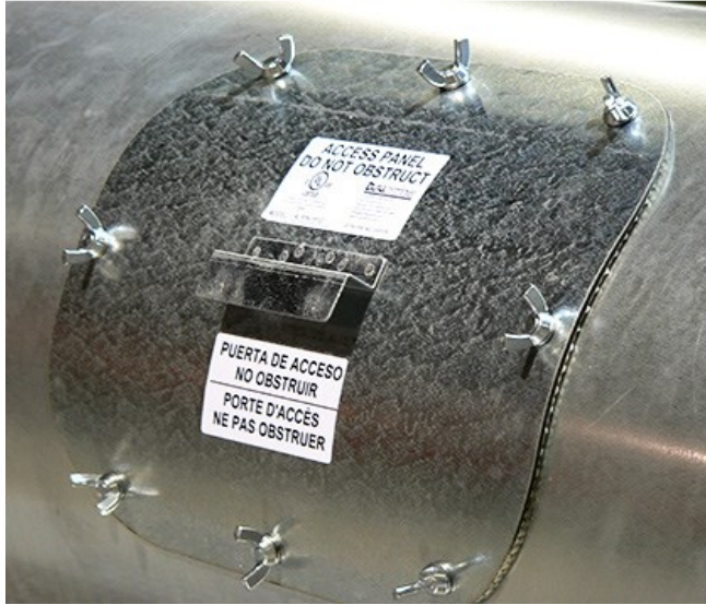
A curved access door installation.
