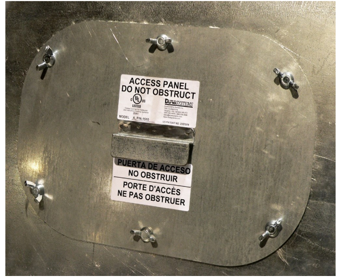
A flat access door installation.
